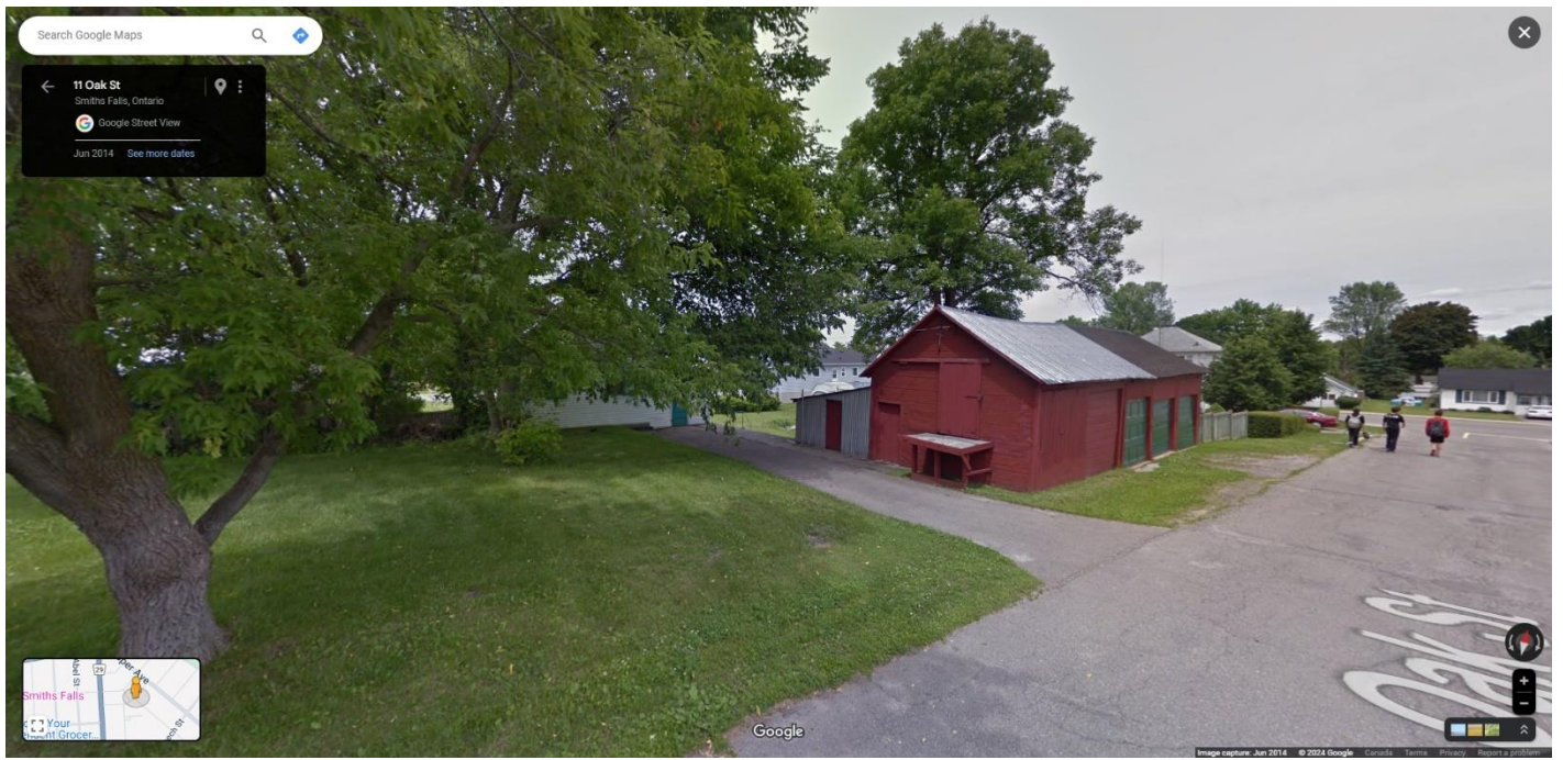
Oak Street View of Subject Property, Courtesy of Google Images (2024), Image Capture, June 2014
