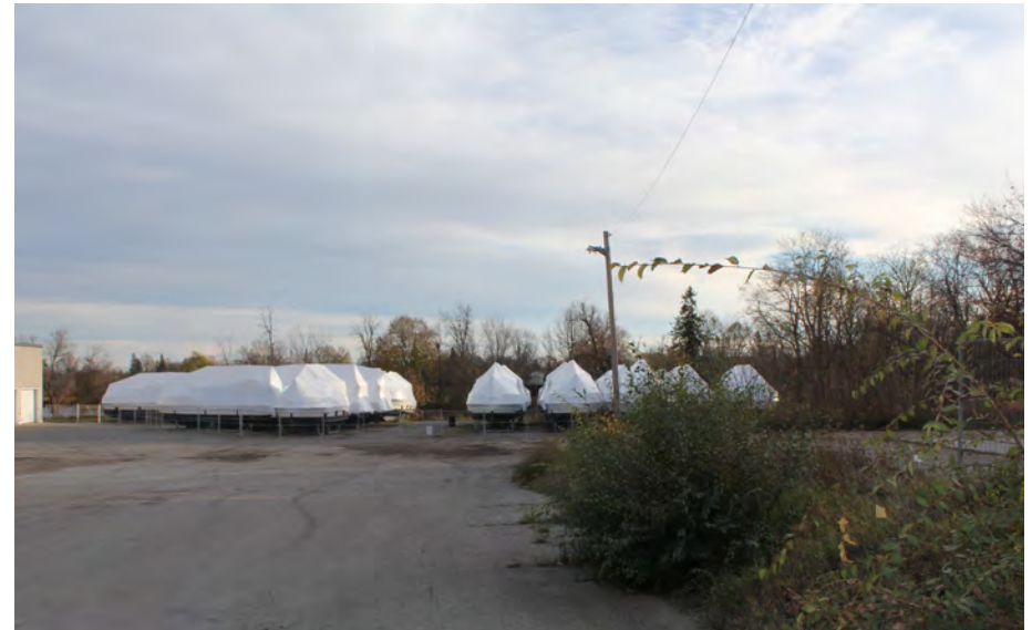
Fig. 16: View of the Le Bout facility. Source: GSP
