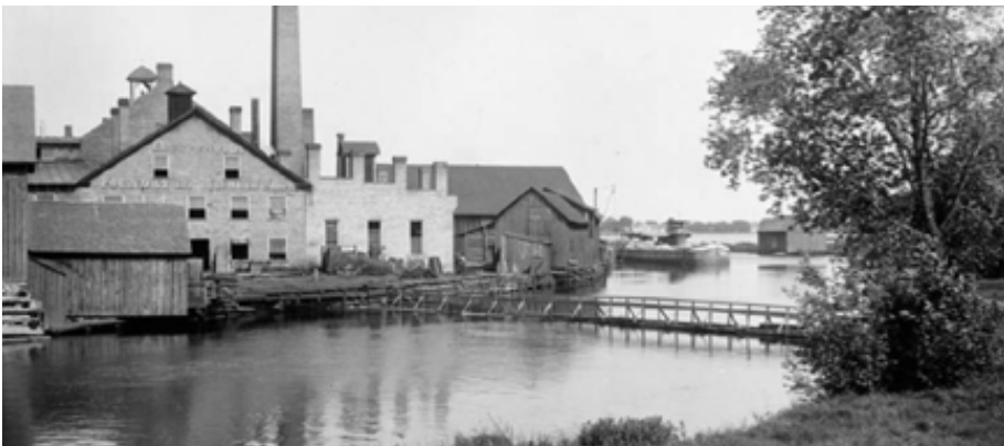
Fig.3: Pedestrian Connection to Frost and Wood across Rideau Canal
