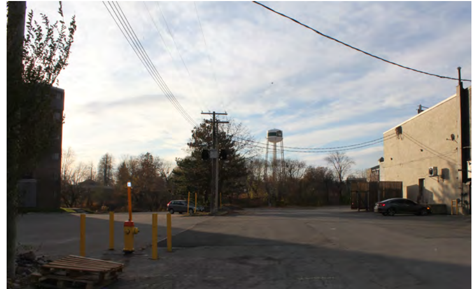
Fig. 15: View of the Smiths Falls water tower from Centre St. Source: GSP
