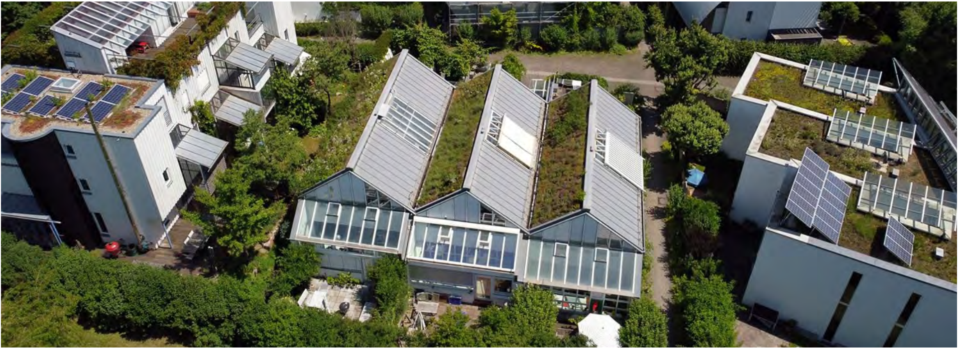
Fig.41: Green Roof and Solar Panel Examples
