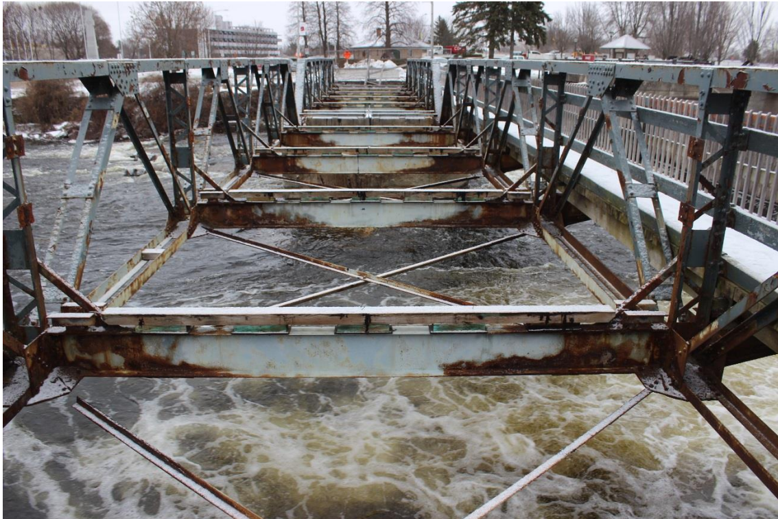
Image 2. Looking east along trusses from west abutment
