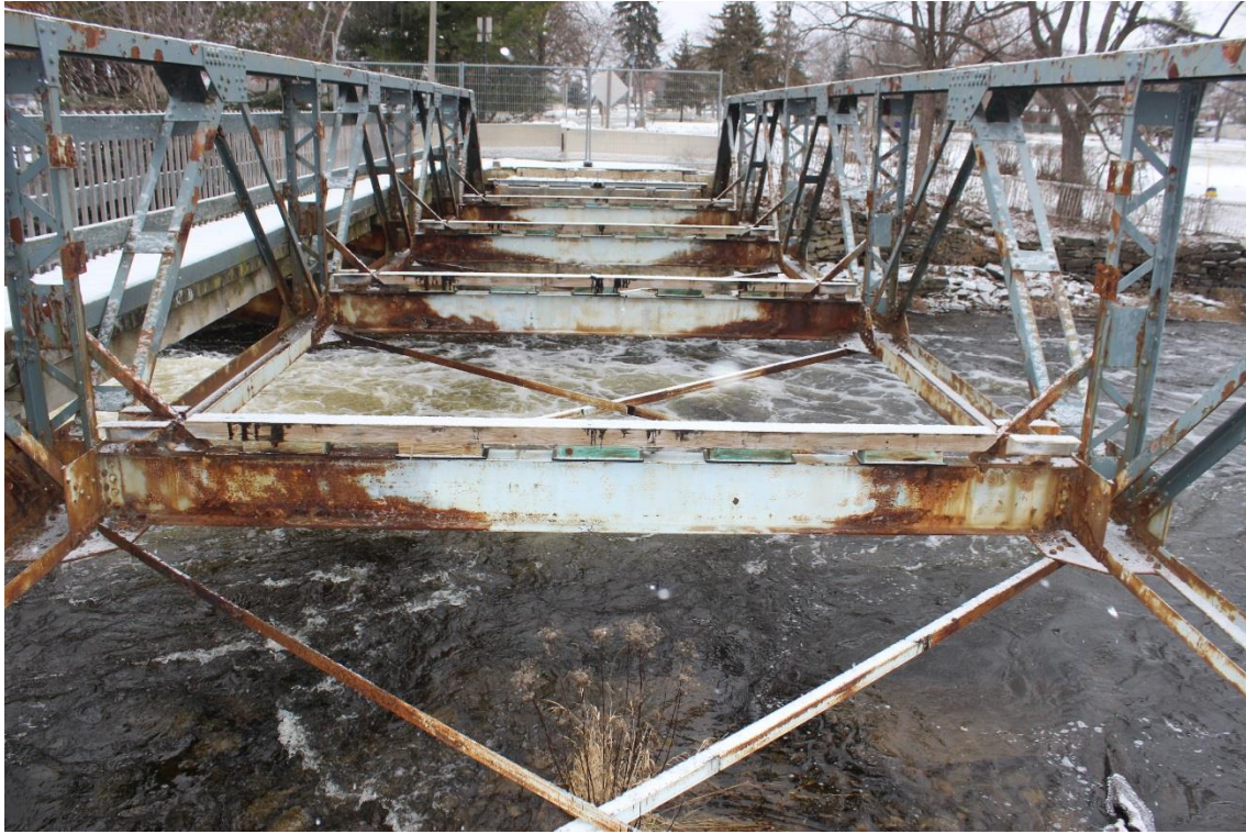
Image 17. West truss viewed from pier
