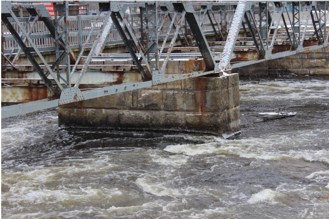
Image 14. East face of pier viewed from east bank
