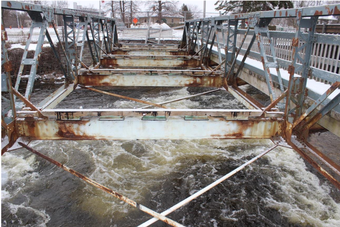
Image 18. East truss viewed from pier
