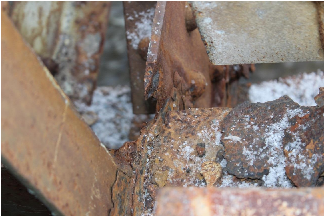
Image 6. East truss panel point 4 upstream perforated gusset plate
