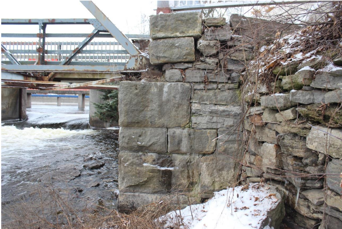
Image 20. West abutment north face
