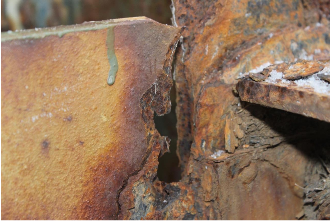
Image 5. East truss panel point 4 upstream perforated gusset plate
