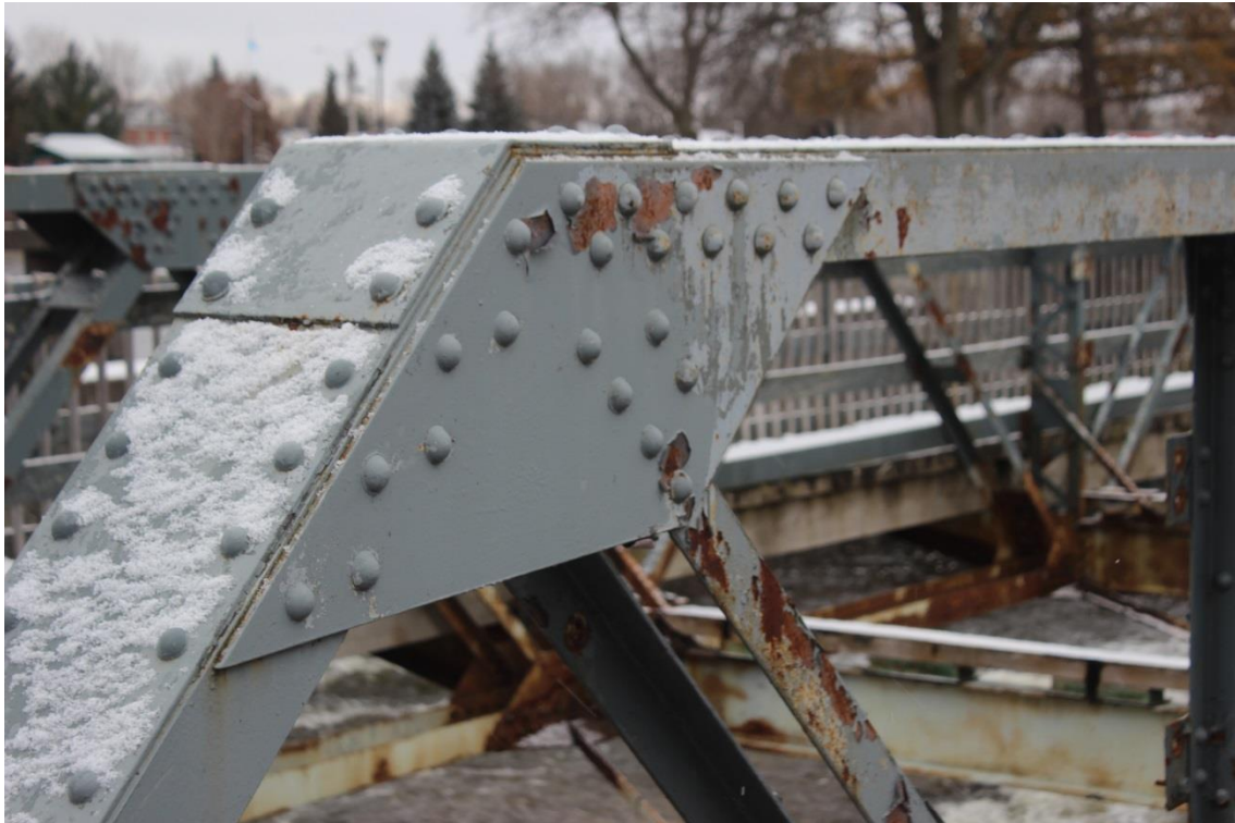
Image 12. Top chord east end gusset of east truss in NE corner
