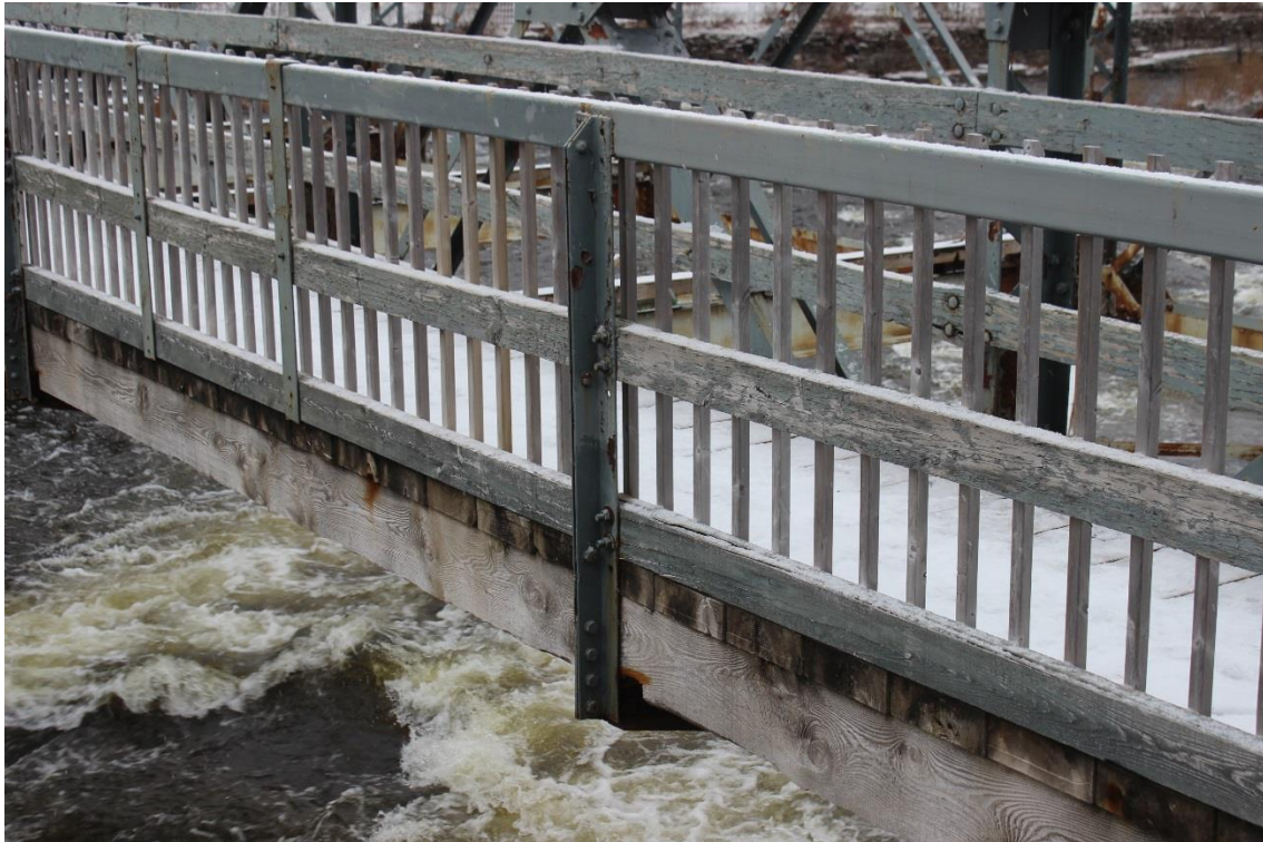
Image 16. Post and railing detail for walkway, east end of east truss
