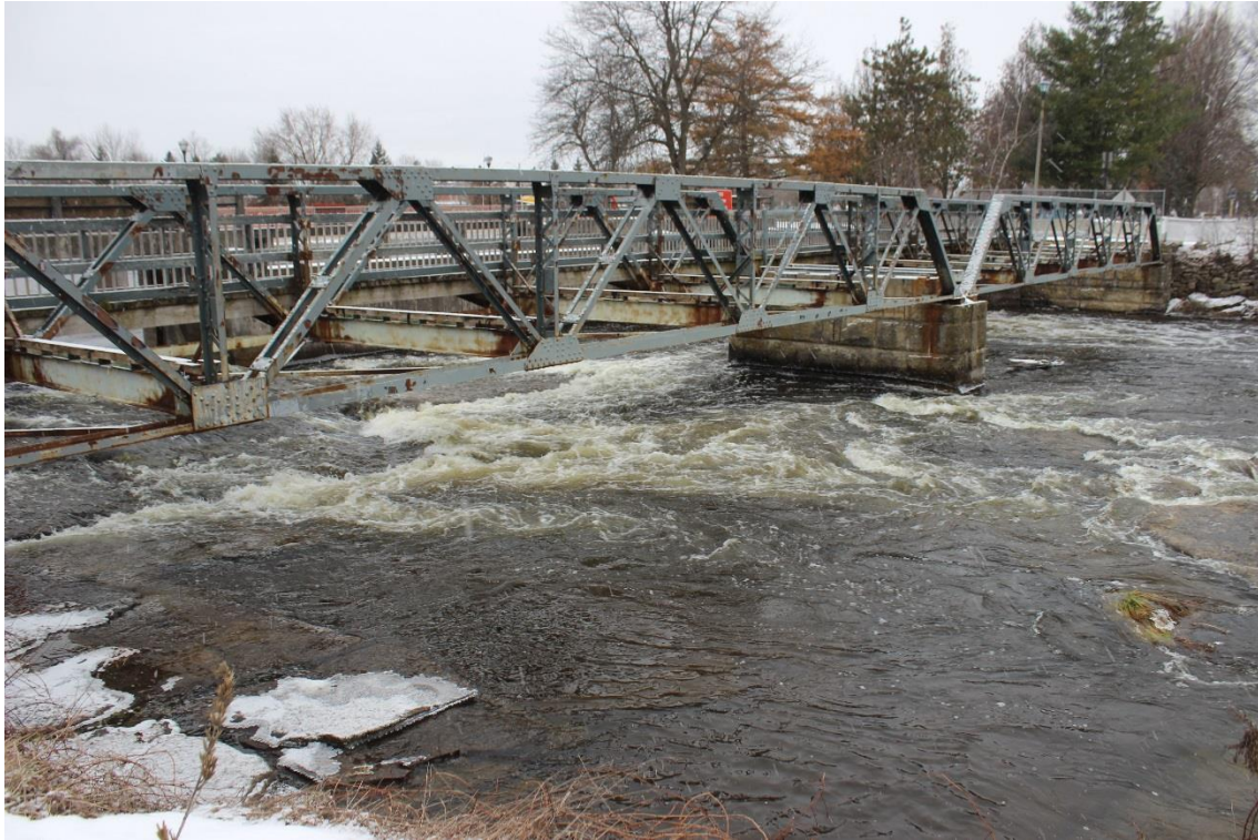
Image 13. Downstream elevation view from east bank
