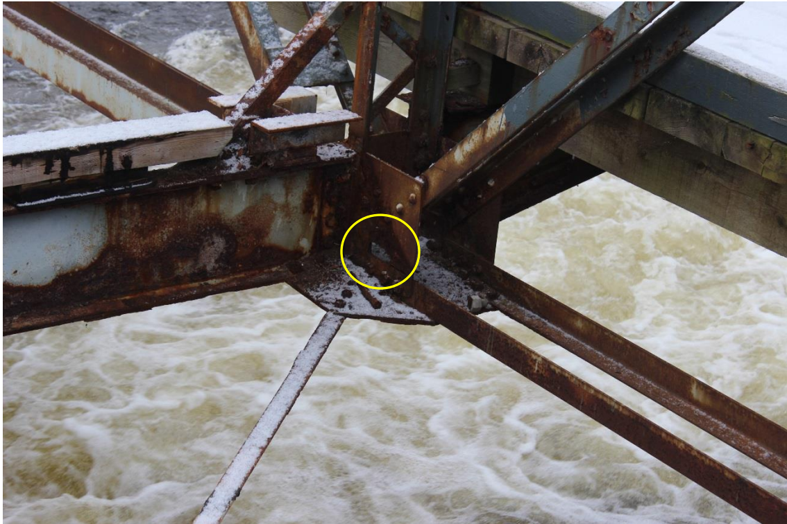
Image 4. West truss panel point 1 upstream perforated gusset plate
