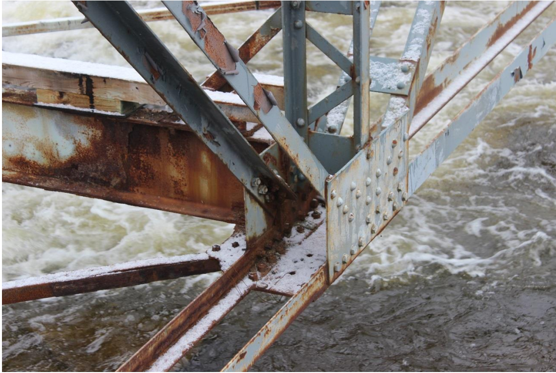
Image 19. Panel point 4, downstream east truss with rivets & high-strength bolts
